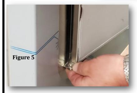
For bottom side remove vice grips/channel locks to access hinge. Repeat step with bushing, rivet and riveter/rivet gun. (Figure 5)
